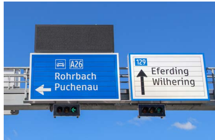
Prism-type variable message signs can display symbols and texts for road closures and alternative routes.
